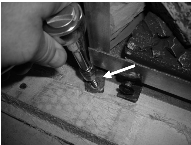
Figure 10 – Shipping Clip Detail
