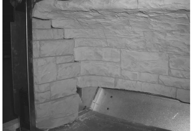
Photo 2 - Left Baffle Panel
