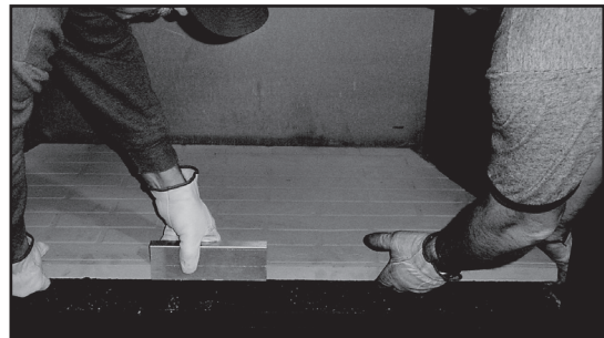
Figure 3.10 Lifting Out Hearth Stone
