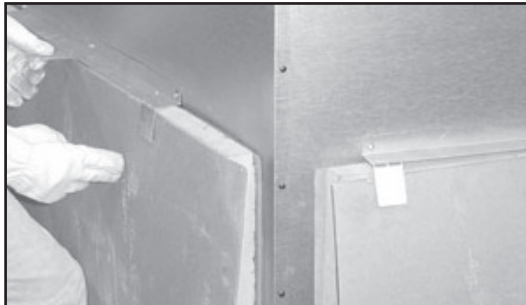
Figure 3.6 Unpack Back Refractory
