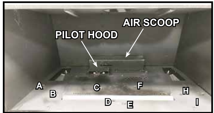
Figure 2. Empty Firebox with Shoulder Screw Locations
