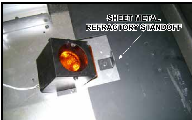
Figure 11.13 Accent Light Bulb Installation Completed
