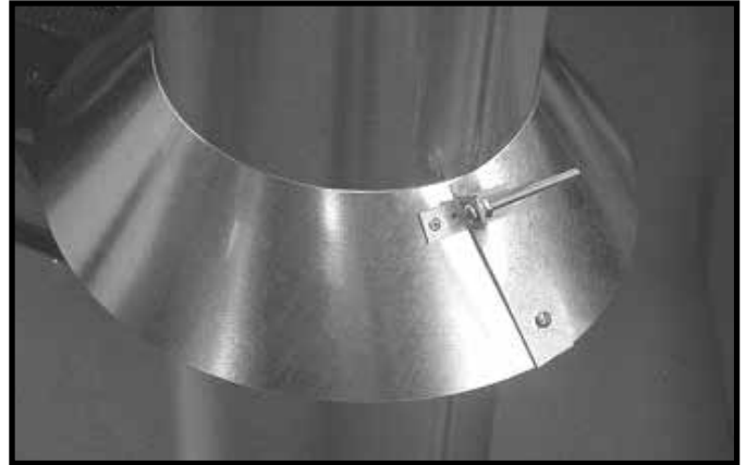
Figure 7.12 Insert Bolt into Brackets
