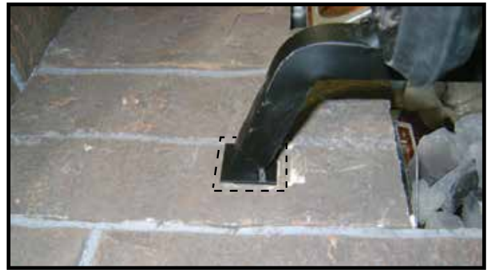
Figure 3. Grate leg placement.
