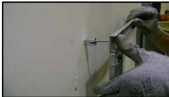
Figure 4.6 Installing Anchors in Hollow Wall
